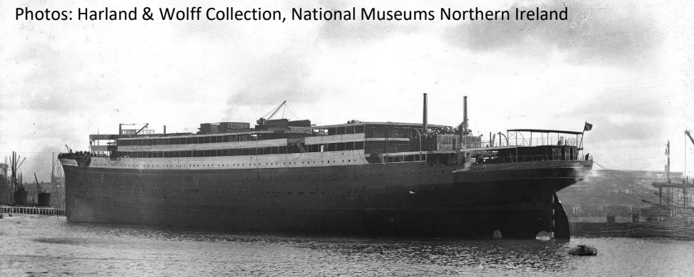
Laurentic enters service on 29 April 1909. The same arrangement of reciprocating and turbine machinery is later fitted to the much larger 'Olympic'-class liners.
