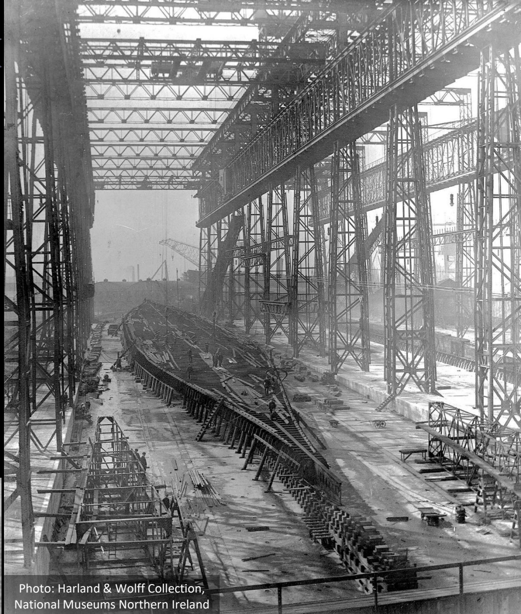
Cross-section of Titanic's double bottom.
